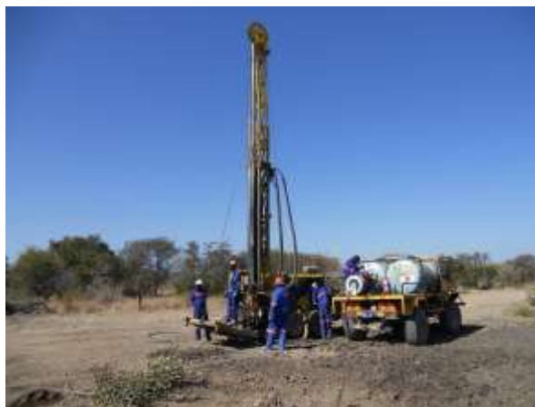
Figure 6: Diamond drill rig
